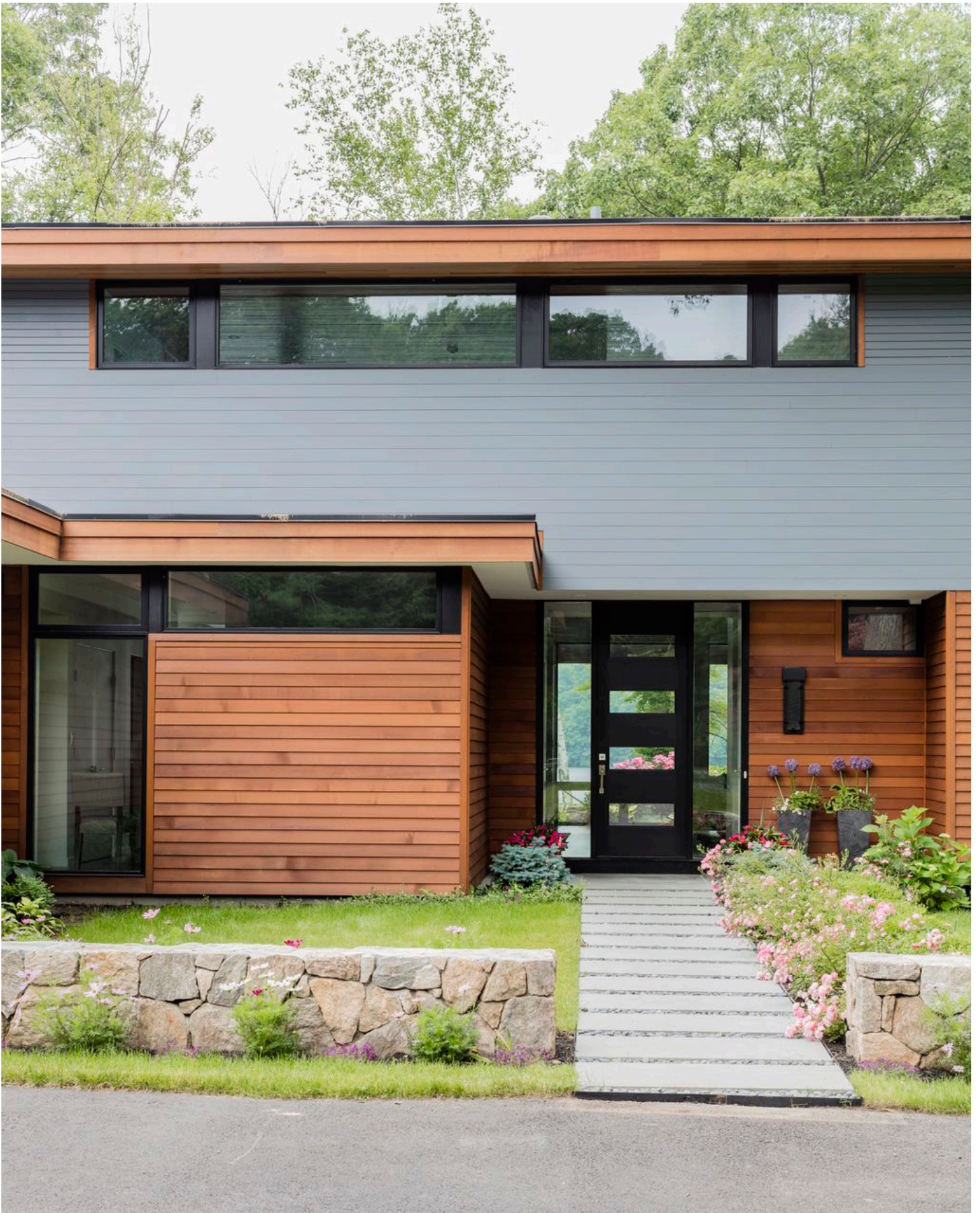
The home by Turkel Design was constructed on site from panelized components, a system that allows for predictability of quality, cost, and timing. MICHAEL J LEE
